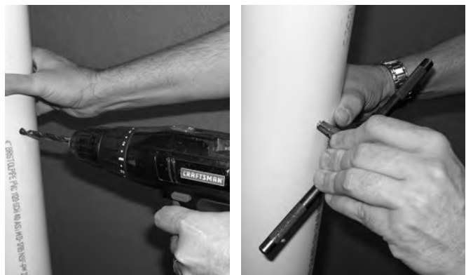
Figure 9.1: Drill and Tap Combustion Test Port
