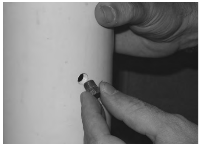
Figure 9.3: Insert Pipe Plug into Test Port
