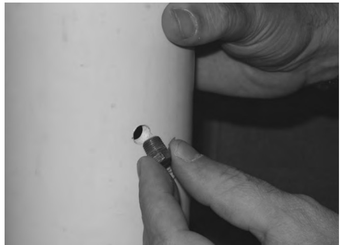
Figure 9.3: Insert Pipe Plug into Test Port
