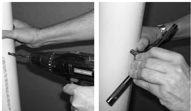
Figure 9.1: Drill and Tap Combustion Test Port
