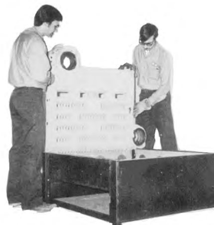
Figure 3.2: Placing the First Section on Base
