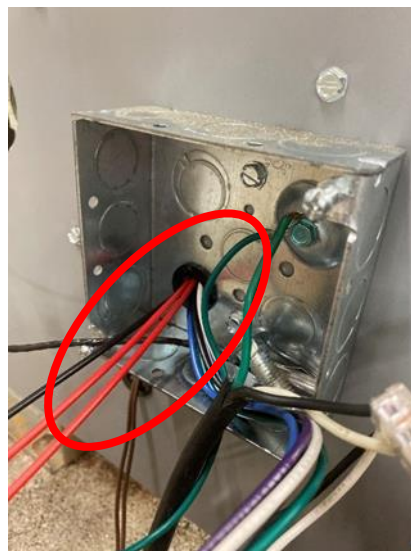
Figure 6: Run wires through hole in junction box
