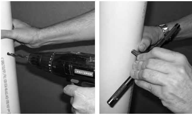
Figure 9.2: Drill and Tap Combustion Test Port
