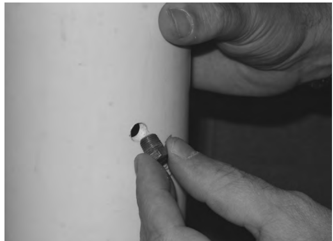
Figure 9.4: Insert Pipe Plug into Test Port
