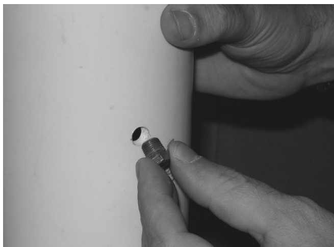
Figure 9.3: Insert Pipe Plug into Test Port
