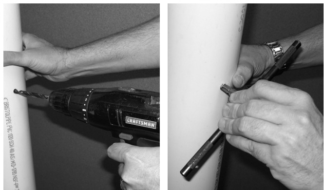
Figure 9.1: Drill and Tap Combustion Test Port
